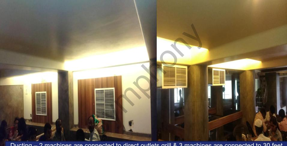
Ducting – 2 machines are connected to direct outlets grill & 3 machines are connected to 30 feet duct having 2 to 3 outlets.
