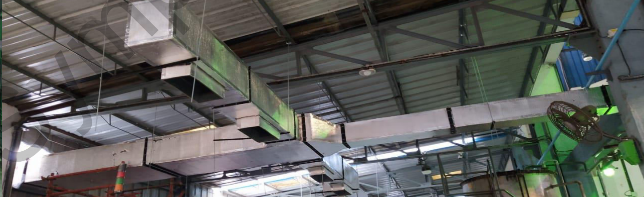
Ducting – All Machines are connected to 45 feet duct having 04 to 05 outlets
