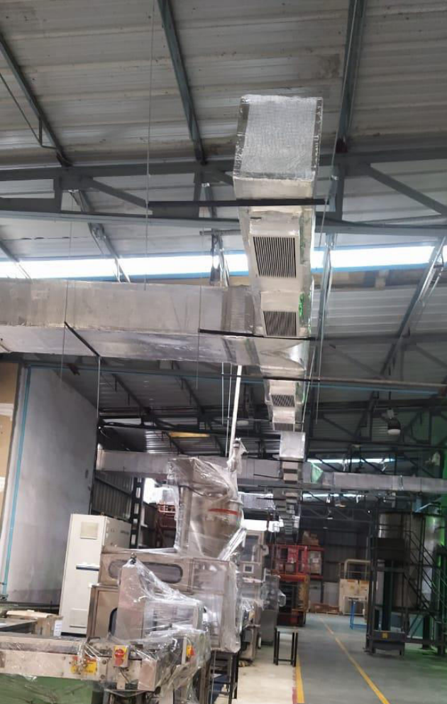
Ducting – All Machines are connected to 45 feet duct having 04 to 05 outlets
