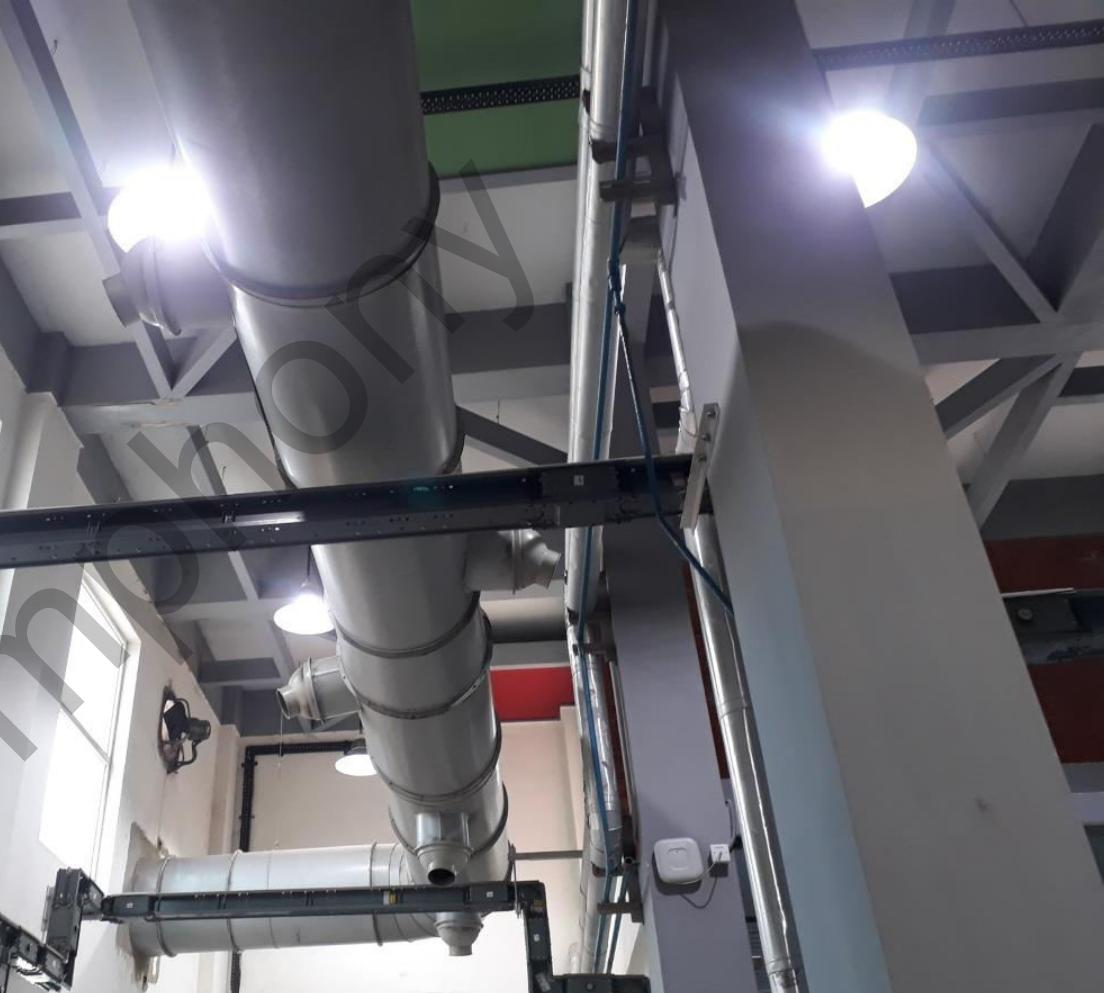
Ducting – All machines are connected to 90 feet duct having 10 outlets
