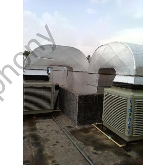
Ducting – All Machine are connected to 30 feet duct having 3 outlets.
