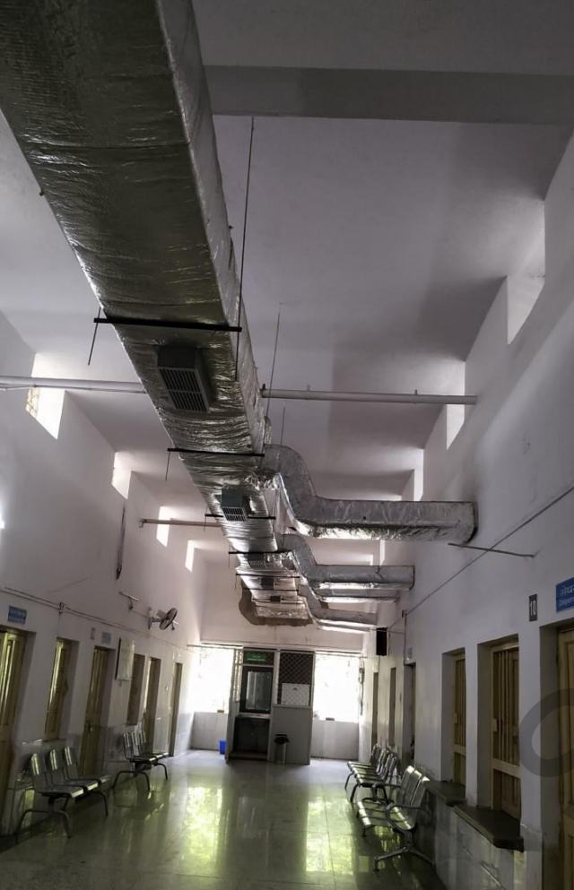
Ducting – All machines are connected to 70 feet duct having 05 to 08 outlets.
