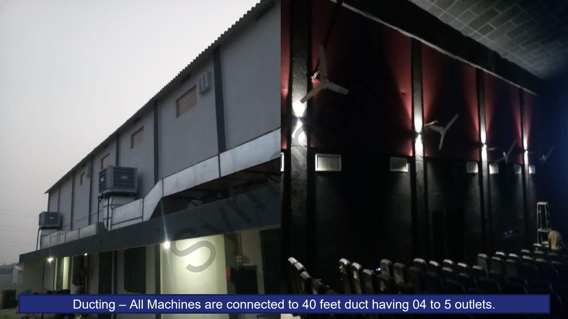
Ducting – All Machines are connected to 40 feet duct having 04 to 5 outlets.
