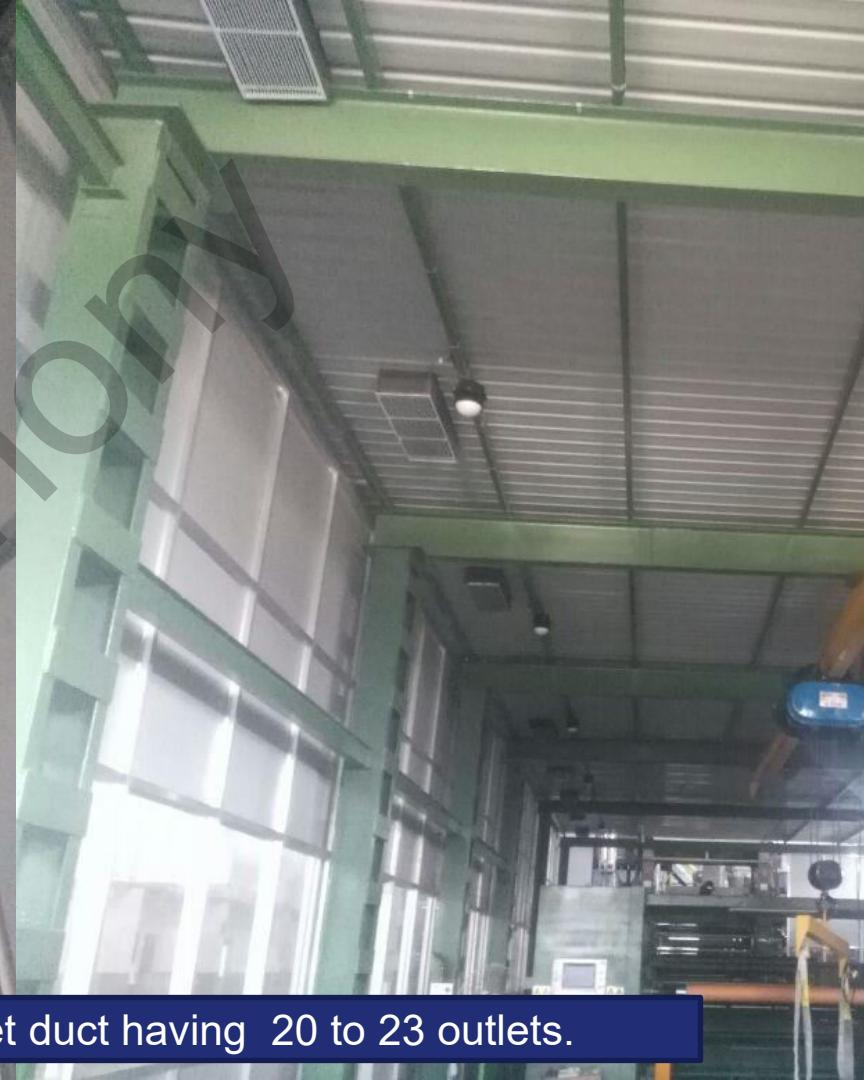
Ducting – Machine is connected to 175 feet duct having 20 to 23 outlets.
