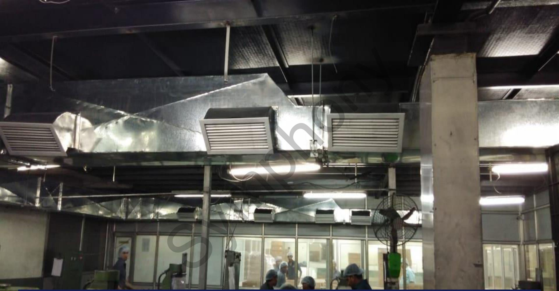
Ducting – All Machines are connected to 70 to 80 feet duct having 12 outlets.
