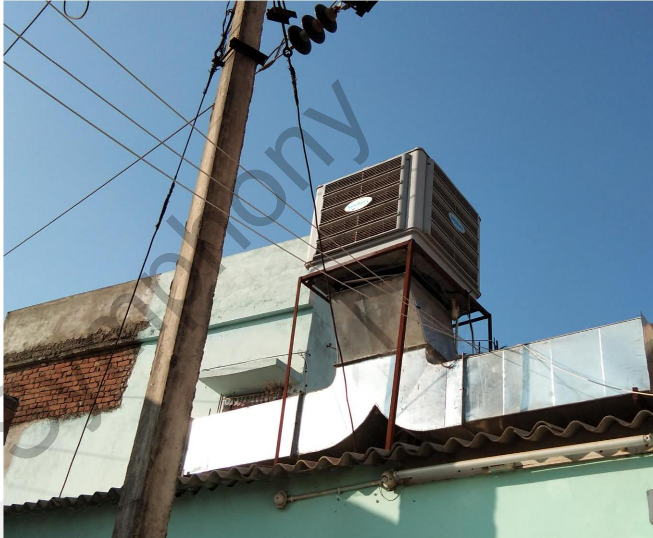
Ducting – Machine is connected to 25 feet duct having 02 outlets.
