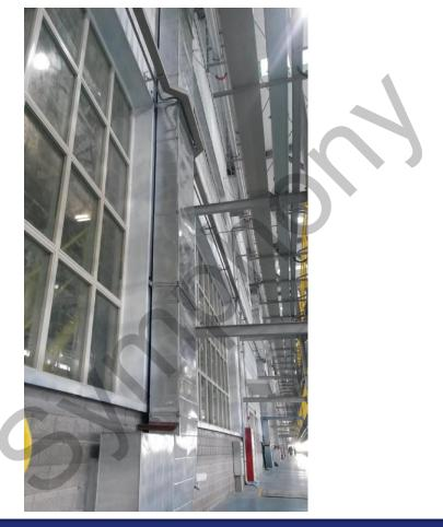
The air pipe is used for direct air supply, and the air outlet adopts aluminium alloy double layer louver air outlet
