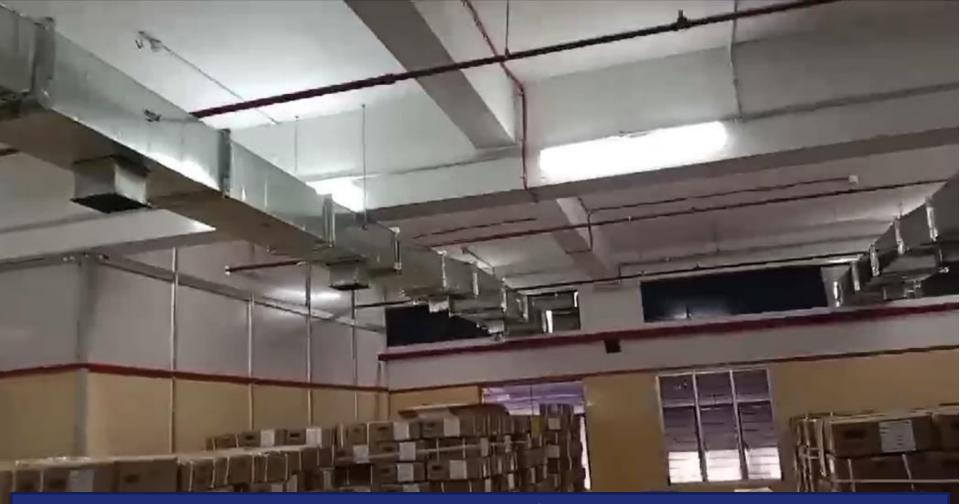
Ducting – All machines are connected to 45 feet duct having 06 to 08 outlets.
