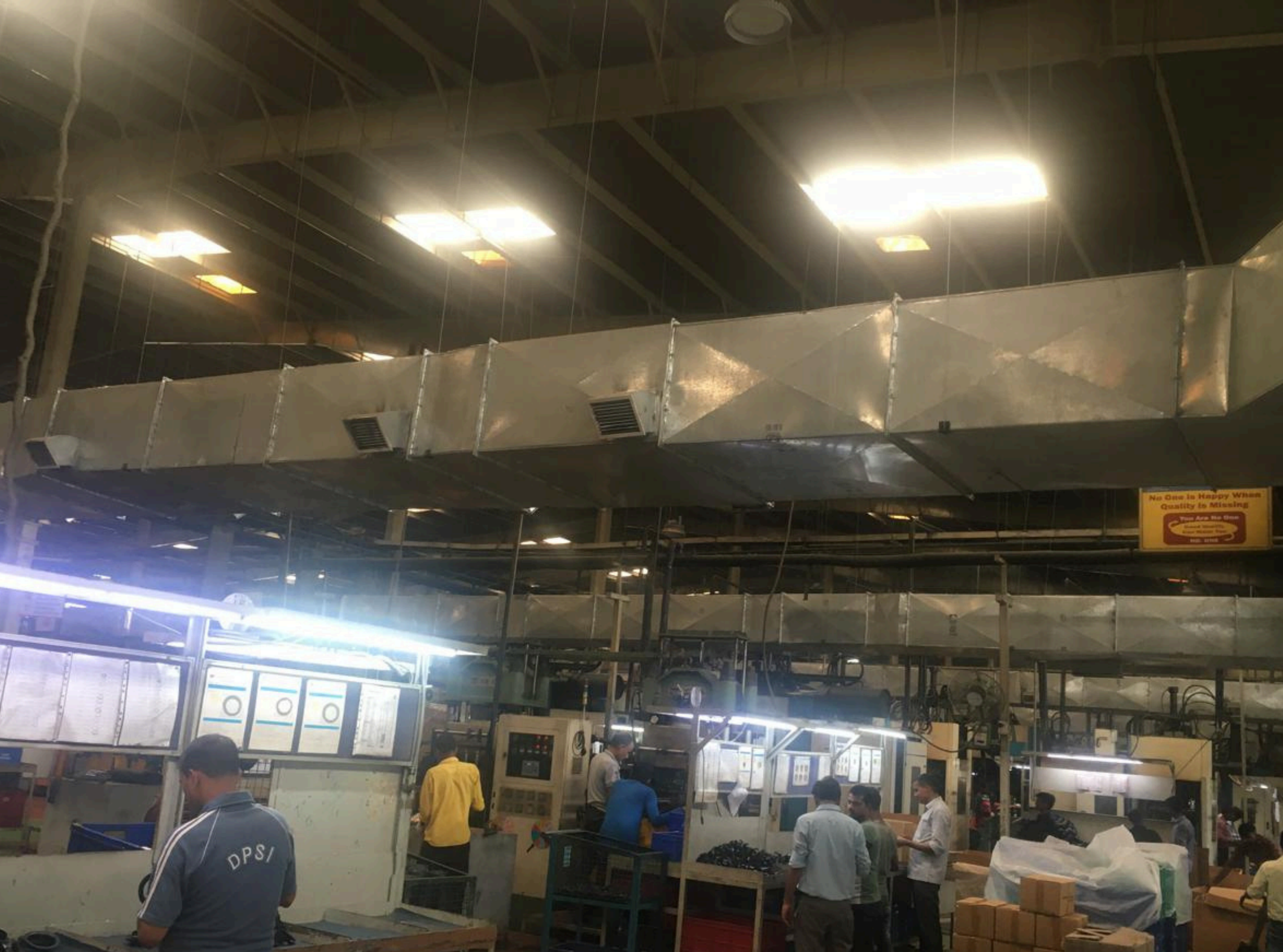
Ducting – 12 Machines are connected to 100 feet duct having 14 outlets
