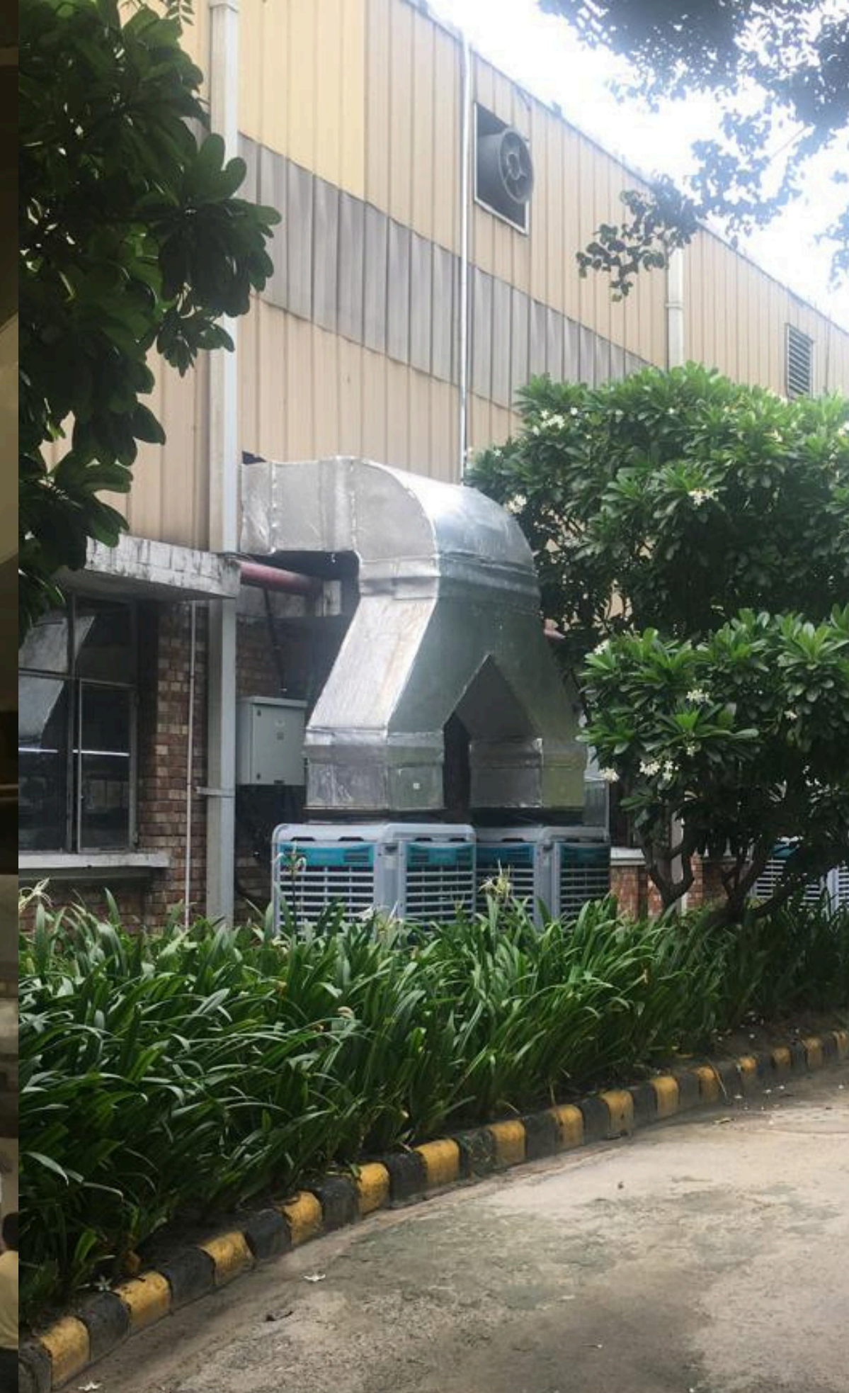
Ducting – 12 Machines are connected to 100 feet duct having 14 outlets
